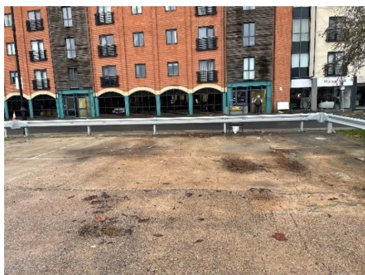
Figure 4 – Worn baylining at Bridge Street
